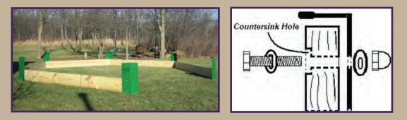
**Attach the bottom layer of boards first** to start the Octagon (or Hexagon) Shape. Attach each board to the brackets, but do not tighten yet. Fit the bolt (with the small washer) through the lumber side at the inside of the countersunk hole. Use the larger washer on the outside of the bracket. Keep the nuts just hand tight for now, as you may need to slightly adjust the position of the brackets to line up the holes on the next layer(s).
