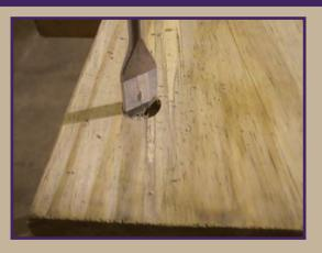
**Once your holes are marked, countersink the marked positions using a 13/16" Spade Bit** (for consistency in depth, mark the bit with a piece of tape at about ¼" above the bottom of the bit body to show your stopping point). Drill the hole until you reach the stopping point marked by the tape. See this step on youtube live at www.youtube.com/watch?v=g3AEsZ2Q9s4
